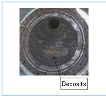
Figure 5 Status of X-6 Penetration entrance before work
