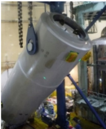
Figure 1 Shielding container for old CI overturned by special crane in CV
