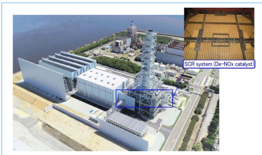
**Figure 1** SCR system for combined cycle power plant demonstration facility at Takasago Works (T-point 2)
