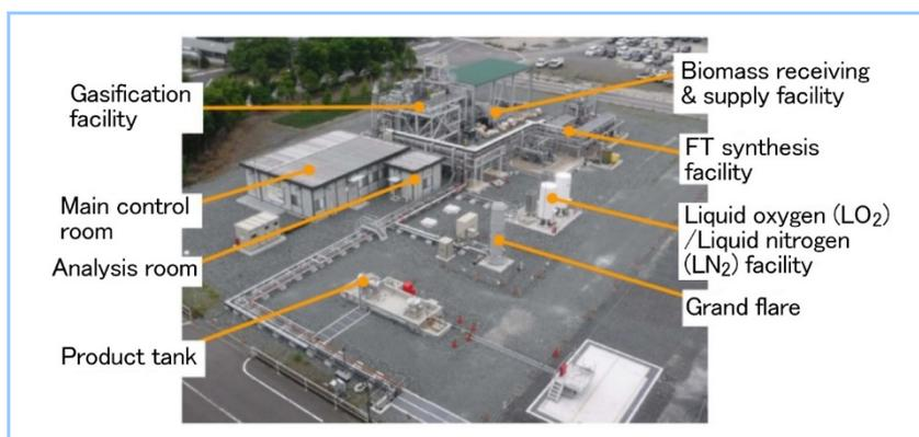
**Figure 6 Full view of the pilot plant**
