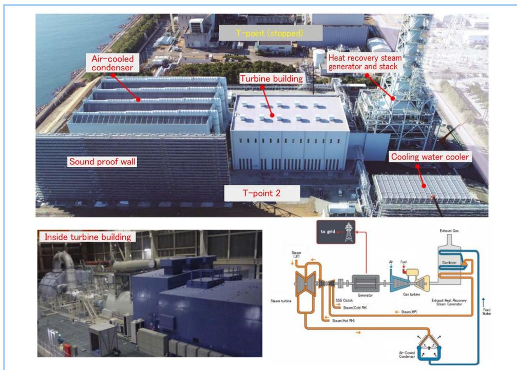
**Figure 5 Overview of T-point 2 combined cycle plan**
