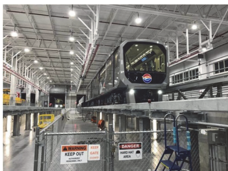
Figure 3 Vehicle maintenance facility
