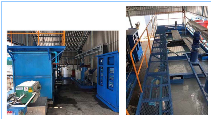
Figure 2 Wastewater treatment plant
