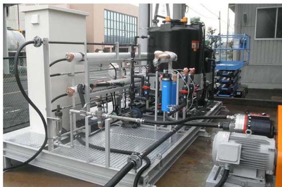
**Figure 7 Exterior of 4-inch RO membrane unit**
