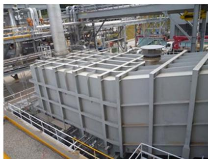
Figure 4 Photo of Los Azufres III Phase I Direct-Contact Condenser
