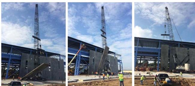
Figure 5 Tilt-wall construction
