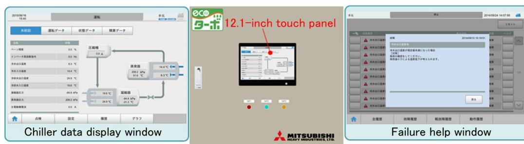
**Figure 2 Appearance and display window of control panel adopting state-of-the-art microcontroller board**
