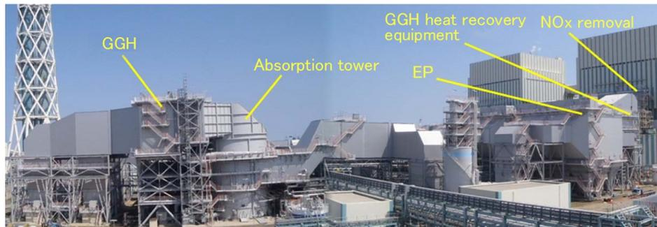
**Figure 3** Exterior view of flue gas treatment facility
