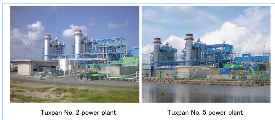
Figure 2 Exterior views of the power plants
