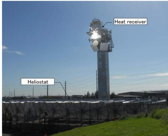
**Figure 5 Verification test of the heat receiver at CSIRO**
