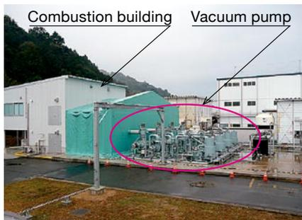
(a) Combustion test facilities
