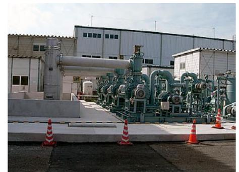
**Fig. 3 Large-capacity vacuum pumps used for the combustion test facilities**
