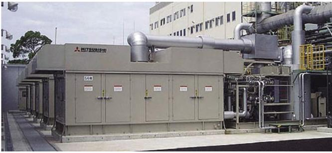
**Fig. 4 The Advanced Miller GS16R-815kW hot water and steam recovery system in operation**
