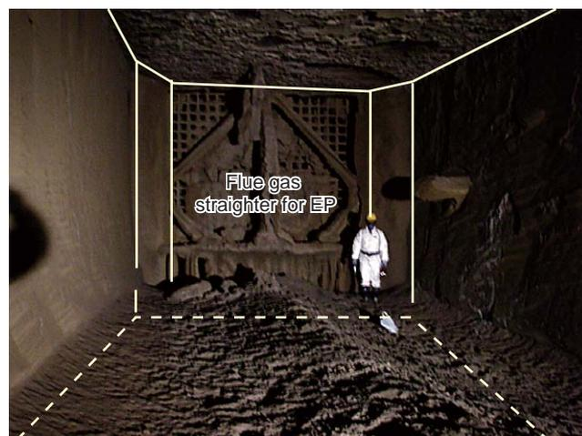
Fig. 15 Ash deposition at the EP inlet flue gas duct
