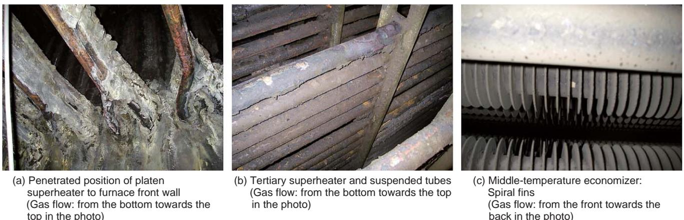
(a) Penetrated position of platen superheater to furnace front wall (Gas flow: from the bottom towards the top in the photo)
