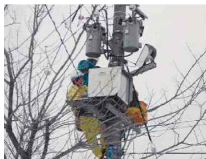
Fig. 6 Camera observation device for lightning strikes
