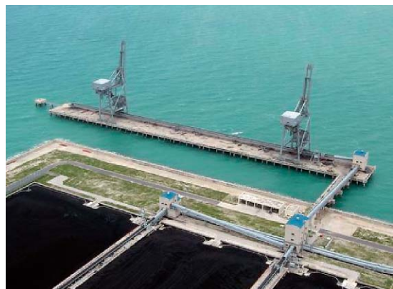
Fig. 9 Coal unloading pier
