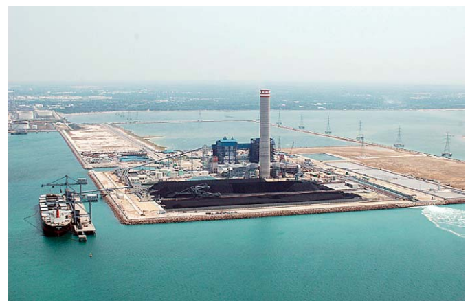
Fig. 2 Overview of the power plant
