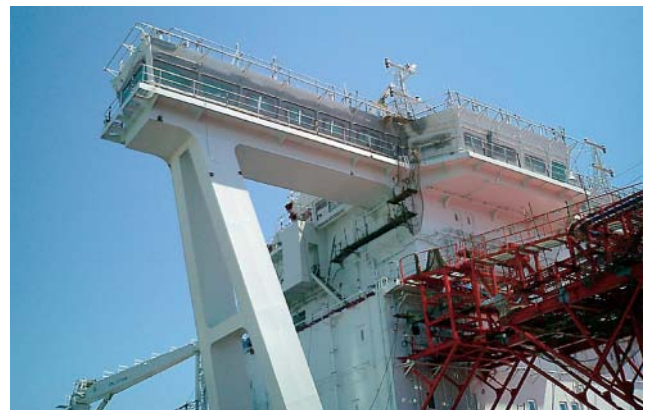
Fig. 5 External appearance of accommodation space of SNOHVIT project ship
