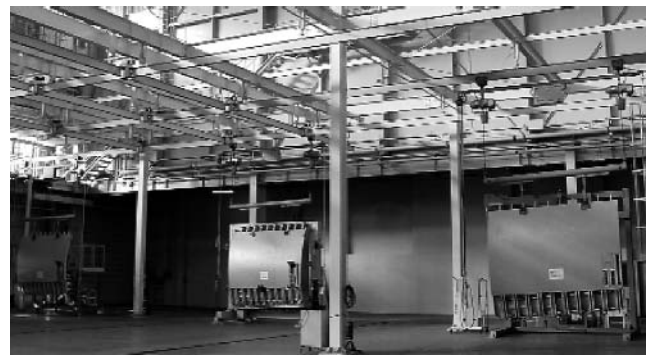
Fig. 4 Monorail Mechanism installation position and dimensional inspection position
