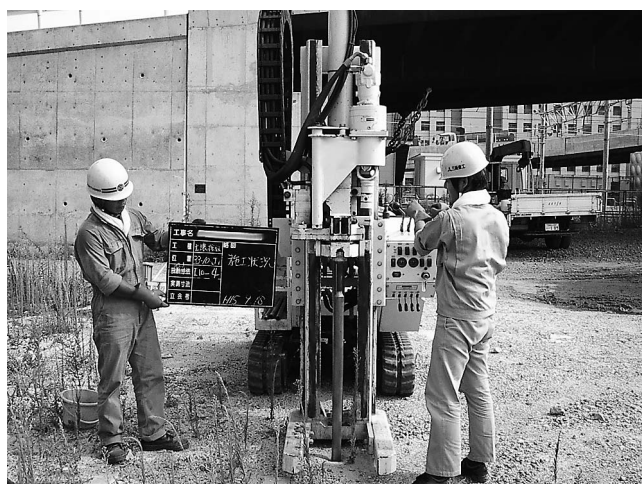
Fig. 1 Self-moving boring machine (Geoprobe)
