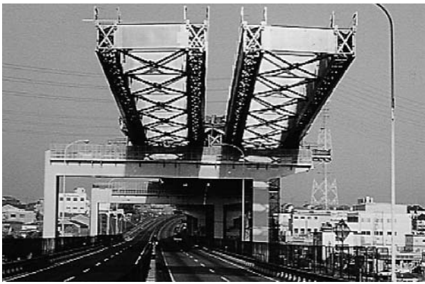
Fig. 9 Rapid launching method
