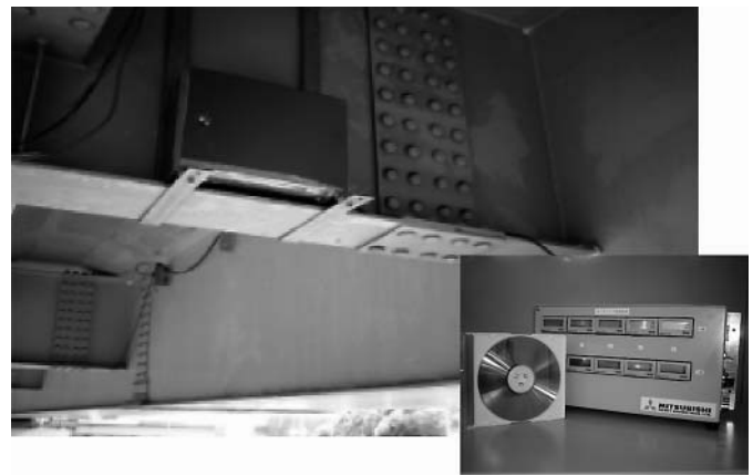
Fig. 8 Fatigue flaw monitoring system
