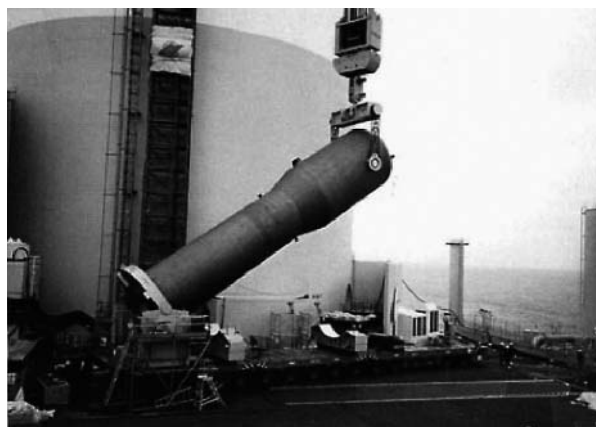
Fig. 13 Steam generator replacement
