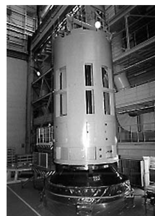
Fig. 14 Reactor vessel head replacement (before shipment)
