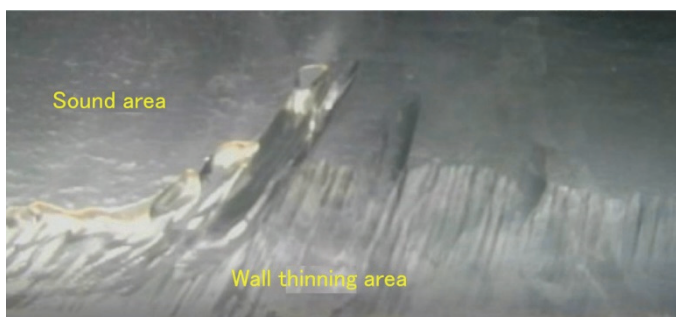
Figure 13 Wall thinning area detected by produced gas piping inspection robot
