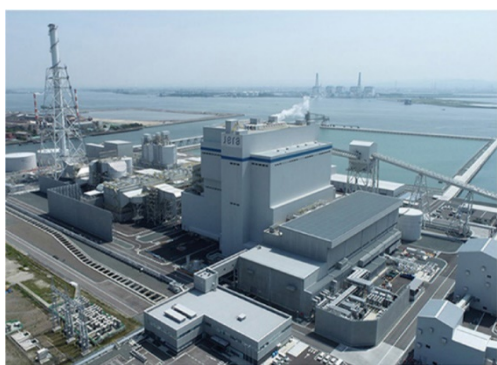
Figure 1 Exterior view of boiler plant (Taketo Unit 5)
