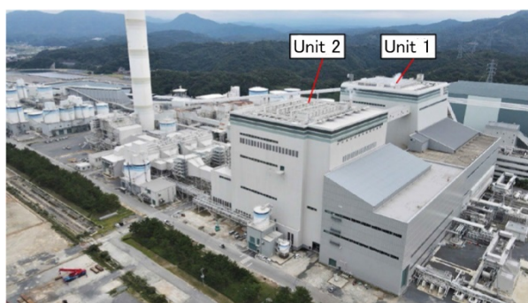
Figure 3 Exterior view of boiler plant (Misumi Unit 2)
