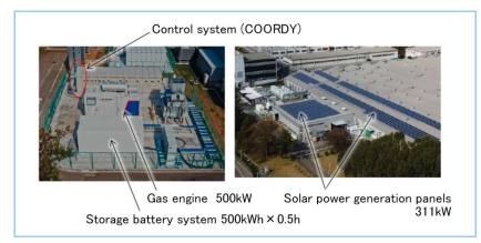
Figure 9 Demonstration facility of hybrid power generation system (EBLOX)
