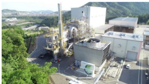
Seifu-shinto Biomass Power Plant (by courtesy of Taihei Dengyo Kaisha, Ltd.)
