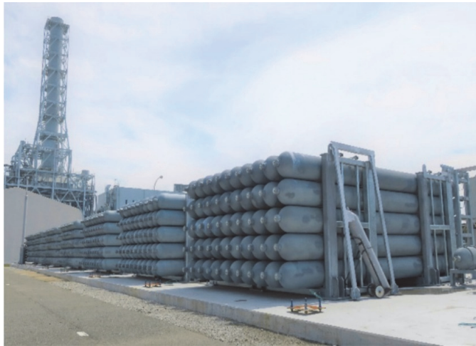
Figure 7 Construction status of Takasago Hydrogen Park (August 2022)
