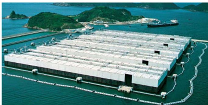
**Figure 2 Large floating marine structure (oil storage facility)**
