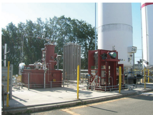
Figure 1 Testing of high-pressure gas safety facility (high-pressure gas production area only)
