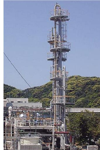
**Fig. 6 Japan CO<sub>2</sub> recovery demonstration plant at a coal-fired power plant**
