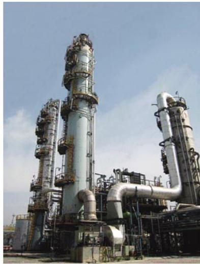
**Fig. 4 India CO<sub>2</sub> recovery plant for urea production**
