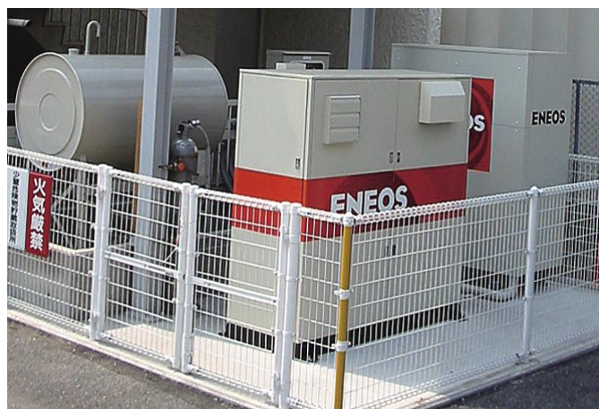
Fig. 4 Kerosene-fueled 10 kW class PEFC system
