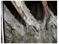
(a) Penetrated position of platen superheater to furnace front wall
