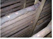
(b) Tertiary superheater and suspended tubes (Gas flow: from the bottom towards the top in the photo)
