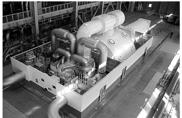
Fig. 1 View of the 600 MW Hirono No.5 steam turbine
