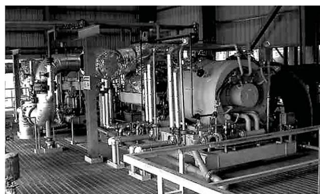
**Fig. 10 On site operation of compressors and steam turbines at a 2 500 tons/day methanol plant**
