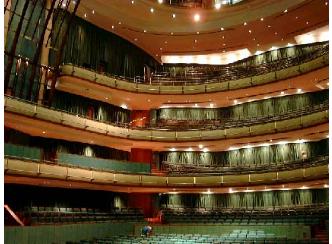
Fig. 5 Acoustic curtain in the Concert Hall
