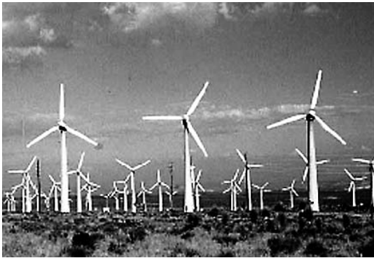
Fig. 4 Tehachapi wind farm in Cal., USA
