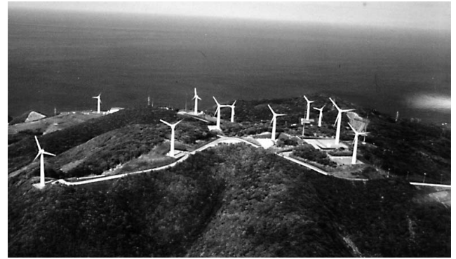
Fig. 5 Tappi Wind Park of Tohoku Electric Power Co., Inc.
