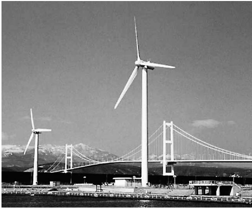
Fig. 3 General view of large-capacity wind turbines
