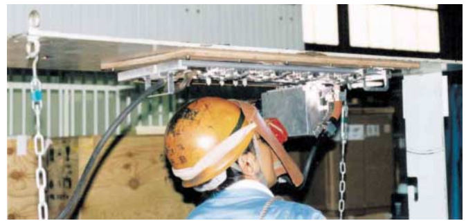
(a) Overhead position welding
