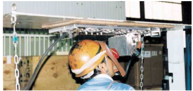
(a) Overhead position welding
