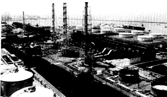
図3 東北電力(株)東新潟火力発電所全景 Higashi Niigata Thermal Power Station, Tohoku Electric Power Co., Inc. A panoramic view of plant
