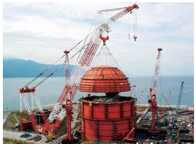
Fig. 6 Large block installation of containment vessel upper head of Tomari Unit 3
