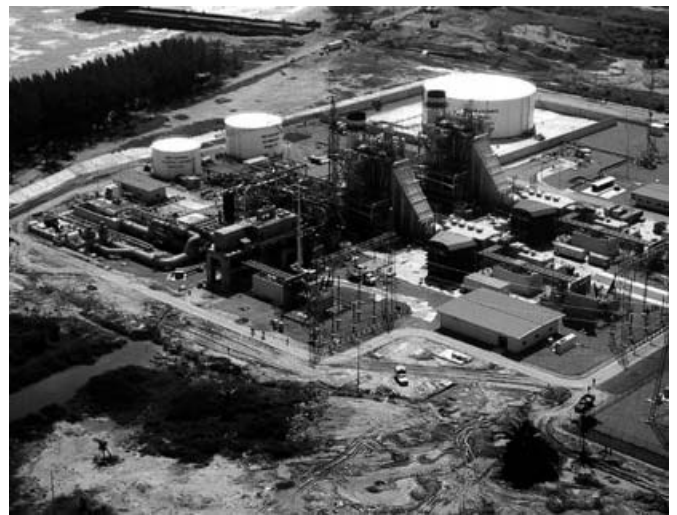
Fig. 5 Tuxpan No. 2 Plant
