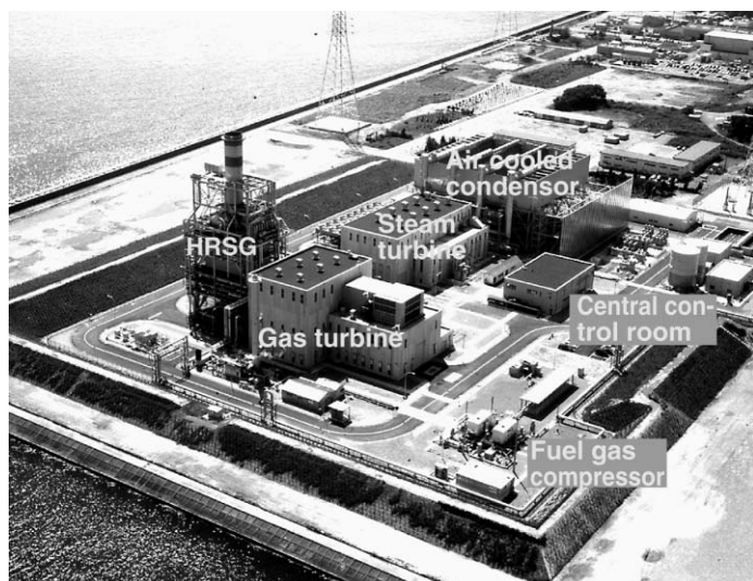
Fig. 2 Gas turbine combined cycle verification plant ("T" point) at Takasago Machinery Works
