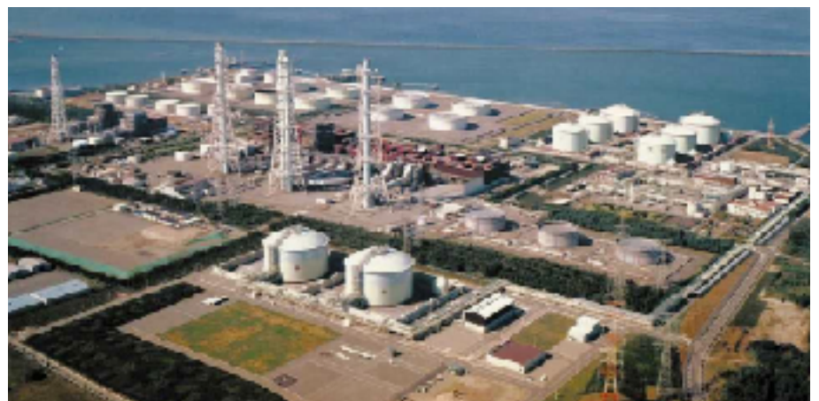
Tohoku Electric / Higashi Niigata No.4, Japan 2on1x1 1999(First), 2on1 x1 (Future)
